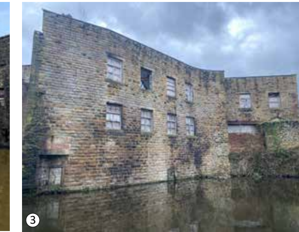
3 Derelict warehouse near Finsley Gate Wharf, Burnley
