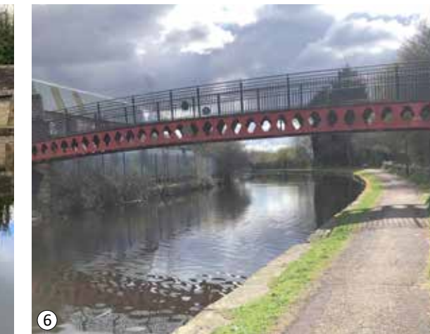
6 Bridge near Blackburn Station
