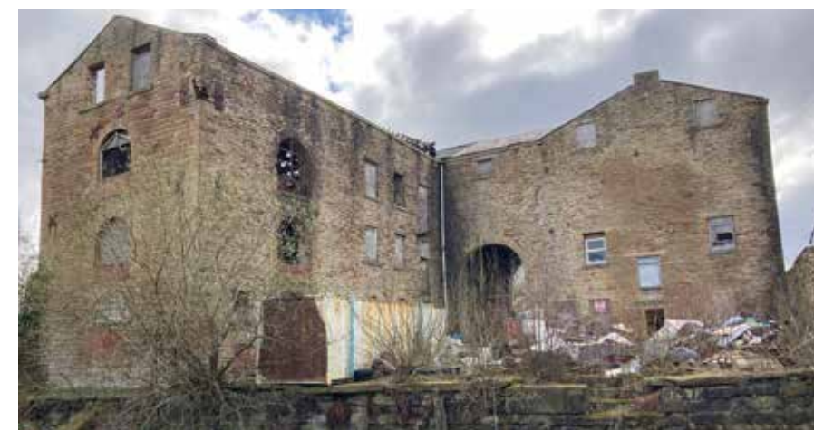
Hargreaves Warehouse, Grade II listed building in a state of dereliction, Church & Oswaldtwistle
