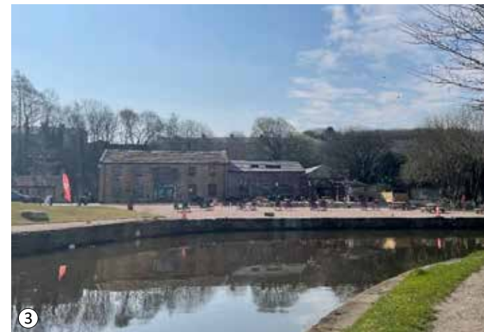
3 Grade II listed Finsley Wharf, Burnley
