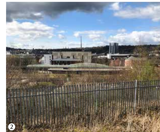
2 View from towpath to industrial area, Blackburn
