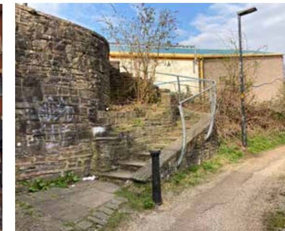
Low level lighting columns adjacent to bridges, Blackburn
