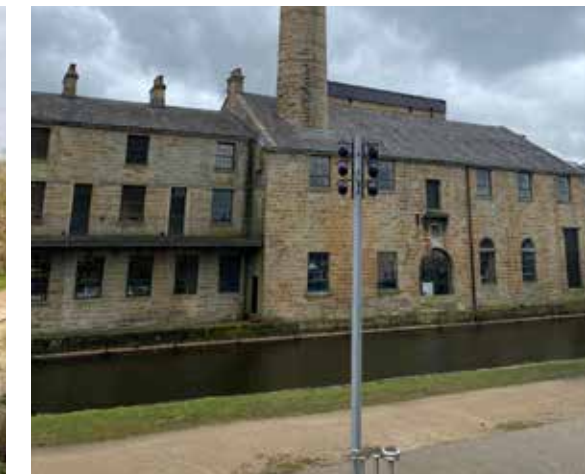
Lighting installation adjacent to Trafalgar Mill, Burnley
