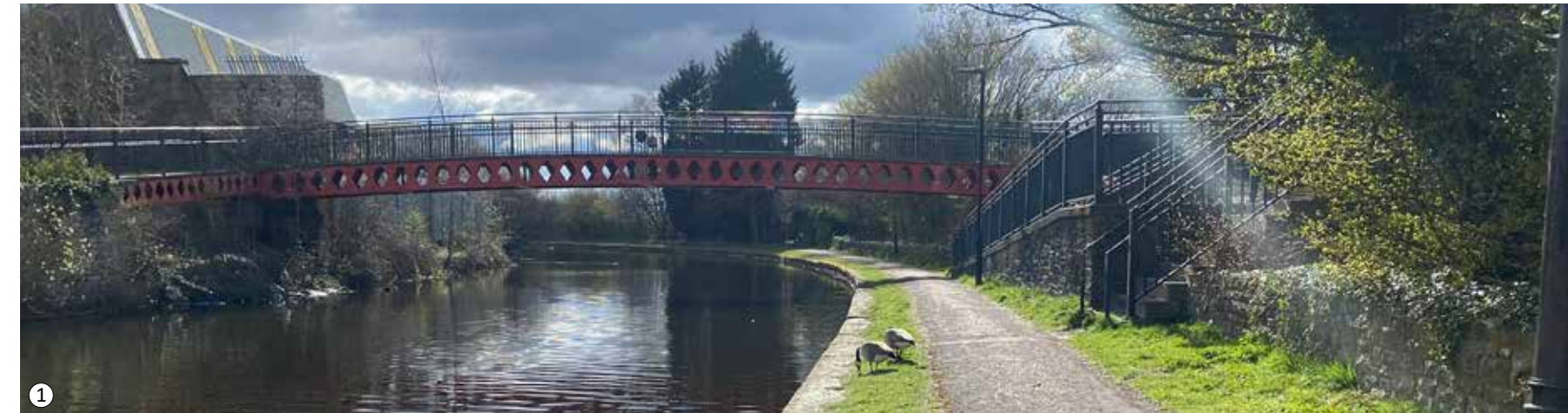
1 View towards pedestrian bridge near Blackburn Station
