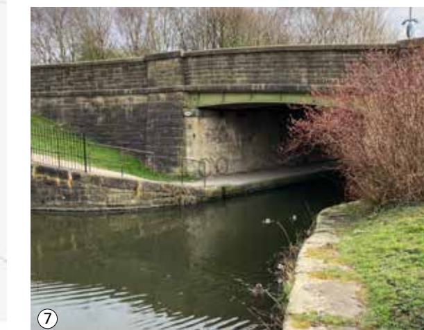
7 Bridge near Enfield Wharf, Hyndburn
