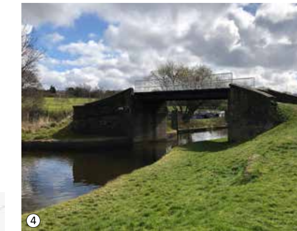
4 Bridge near Reedley Marina, Pendle
