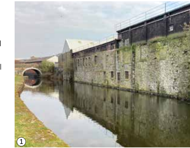
1 Facades/ Walls near Blackburn Station
