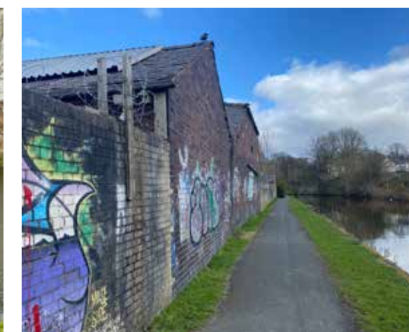
Industrial buildings backing onto the canal, Burnley
