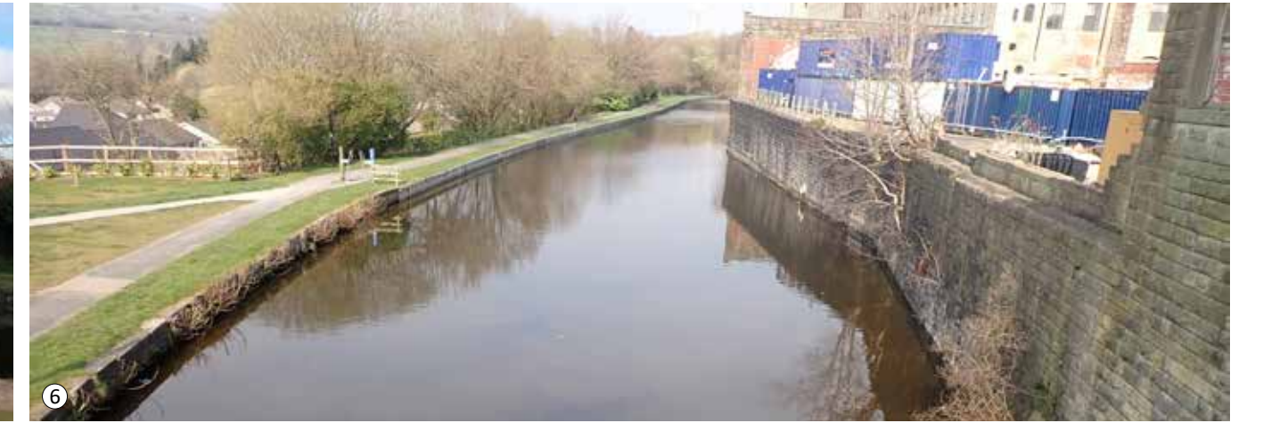
6 View from the bridge crossing towards Northlight and the adjoining walls, Brierfield
