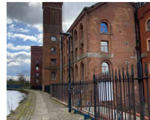
Low level lighting columns along the Blackburn towpath
