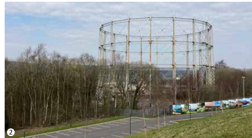
2 View towards the Brierfield Gas holder close to Northlight
