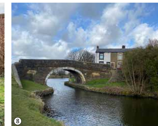
8 Grade II listed bridge, Church Kirk Bridge, Hyndburn
