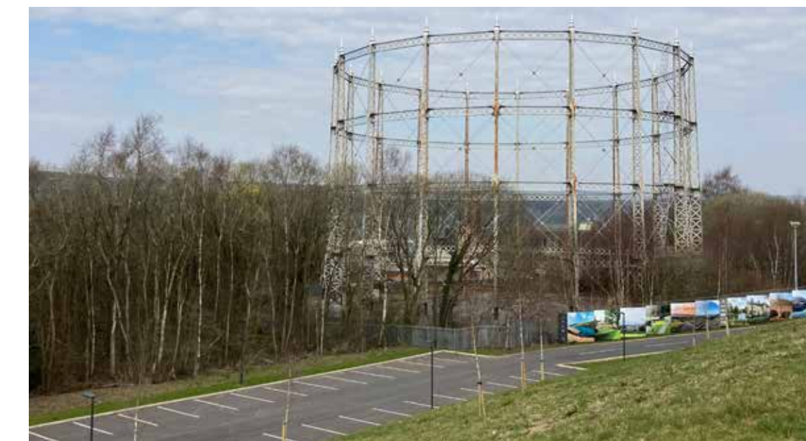
View towards the Brierfield Gasholder close to Northlight
