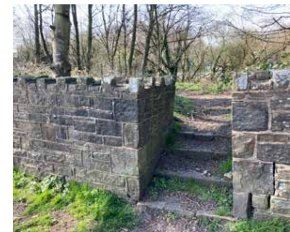
Stepped access to Thompson Park, Burnley
