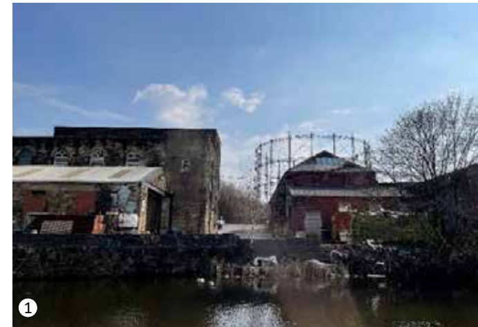
1 Brierfield Gasholder, Pendle
