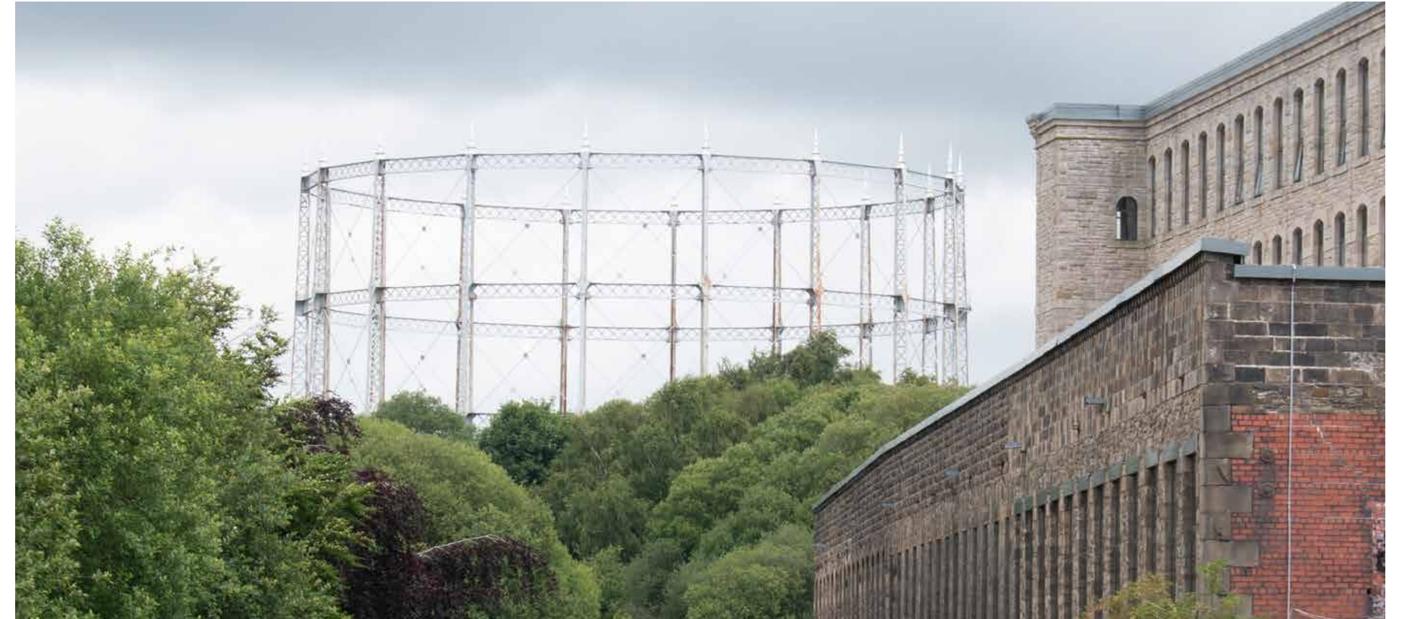
Northlight in the foreground and the Brierfield Gasholder in the background, Pendle
